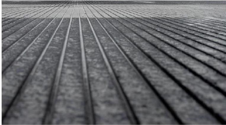
**Figure A6-4. Grooving of asphalt surface
