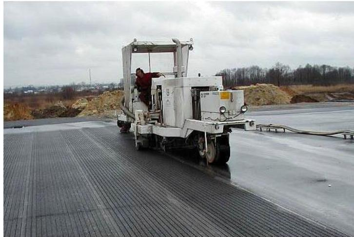
**Figure A6-5. Grooving with saws**
