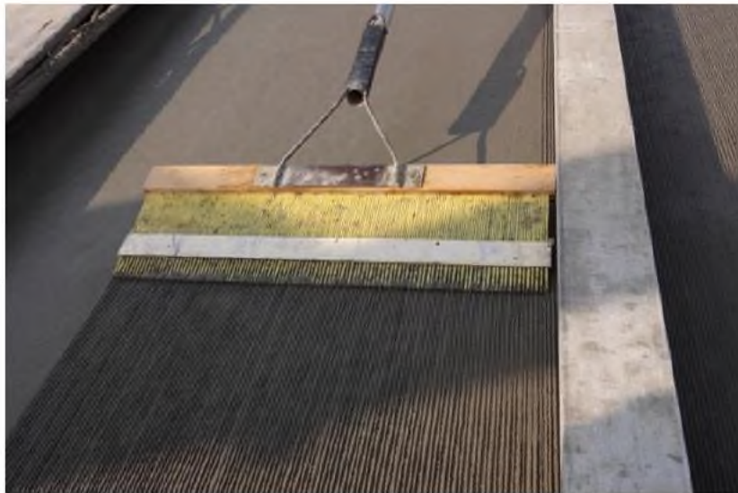
Figure A6-6. New concrete surfacing textured with wire comb
