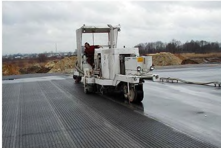
Figure A6-5. Grooving with saws
