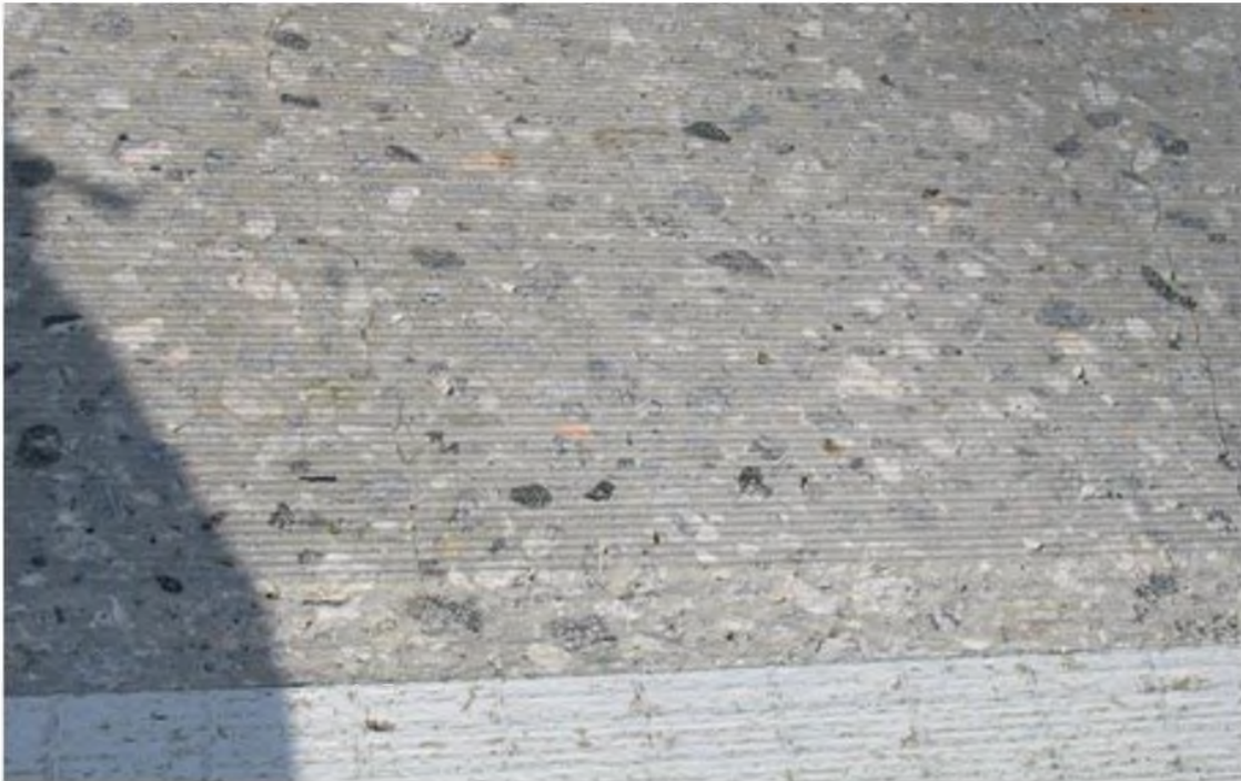
Figure A6-7. Existing Portland cement concrete (PCC) before and after grinding
