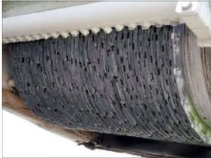
Figure A6-8. Diamond grinding of cement concrete
